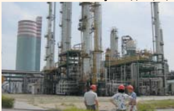
External view of the Inner Mongolia Fertilizer Plant
