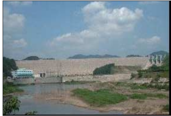
Site Photo: Imha Multipurpose Dam
