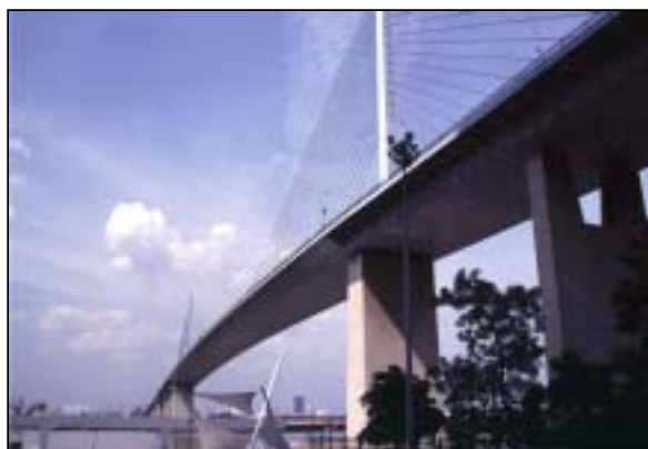
Site Photo: The bridge section of the Chao Phya River crossing
