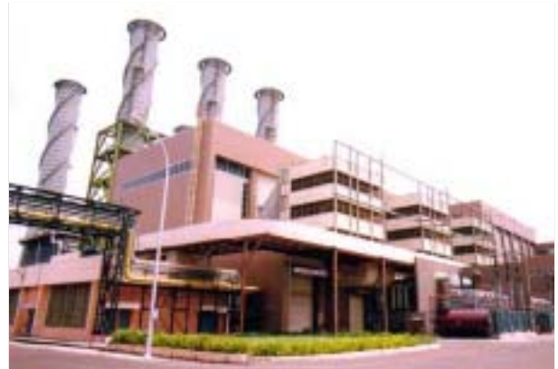
Gandhar Gas Based Combined Cycle Power Plant
