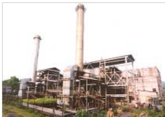
Chandrapur Thermal Power Station
