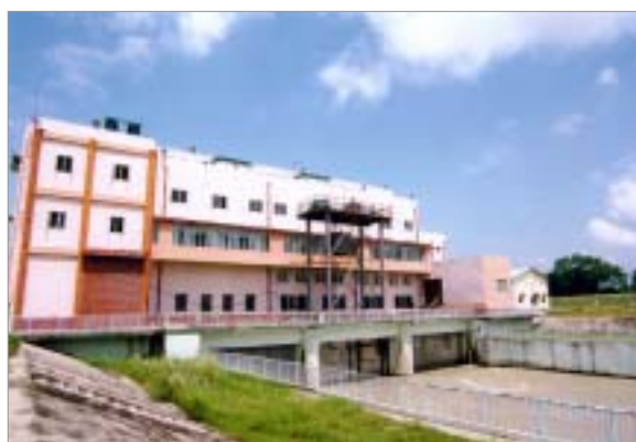
Teesta Canal Hydroelectric Power Station No.3
