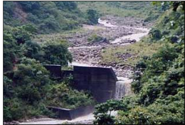
Site Photo : Sabo dam on the Kani River
