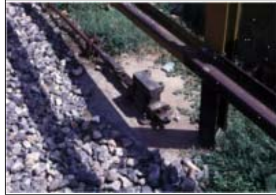
Site Photo: Dina Station
