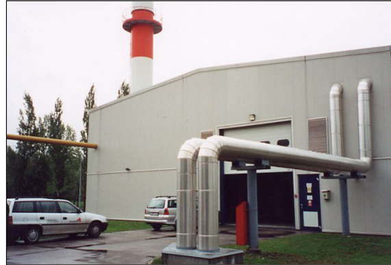
Site Photo: Heating Power Plant (Varpalota)
