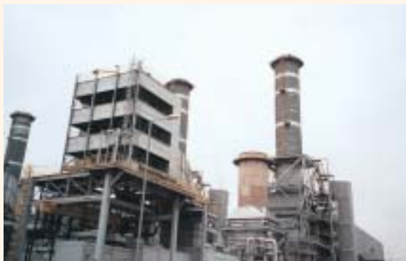
Jandar combined cycle power plant
