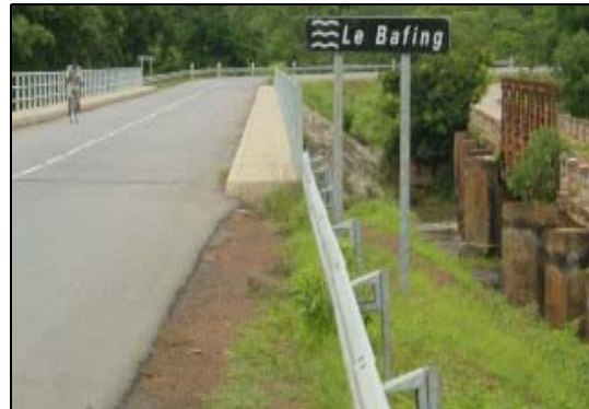
Site Picture (Bridge and Road)
