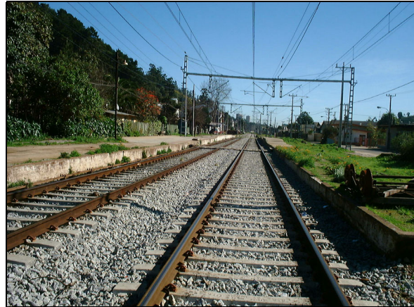
Site Photo: Track and Contact Lines After Renovation (Valparaiso)
