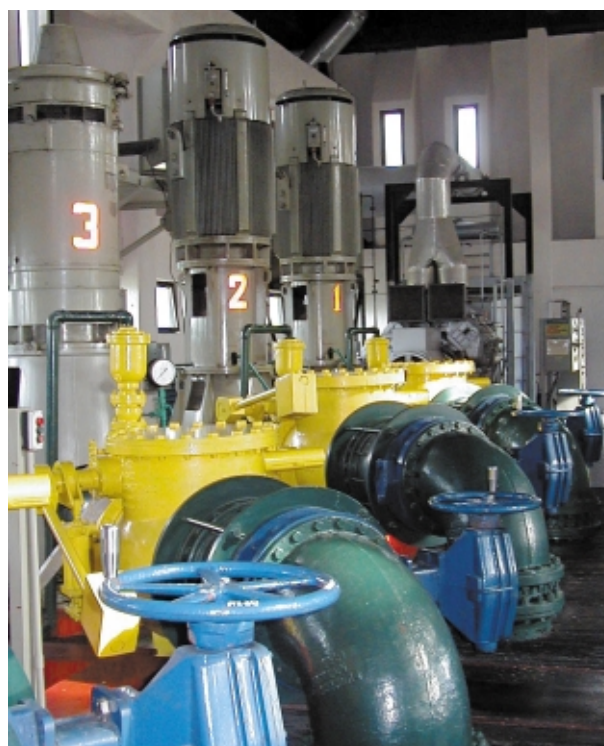
Pump station up using Japan's ODA loan
