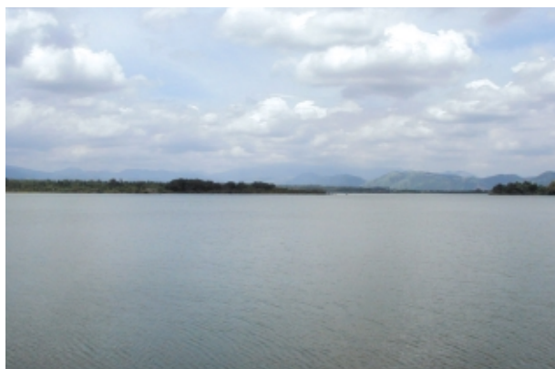
La Mesa Dam located in the northern area of Metro Manila
