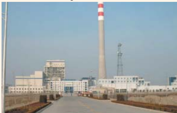
Sanhe Power Plant constructed via the project
