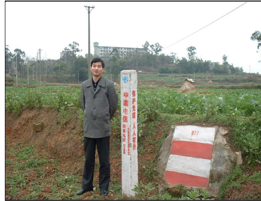
Marker pole at the site where the optic cable is buried (Huayangzhen, Shangliu County, Chengdu, Sichuan Province)
