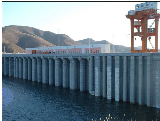
Baishi Multipurpose Dam sluice gate
