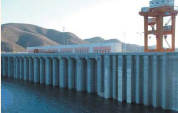
The Baishi Multipurpose Reservoir constructed by this project
