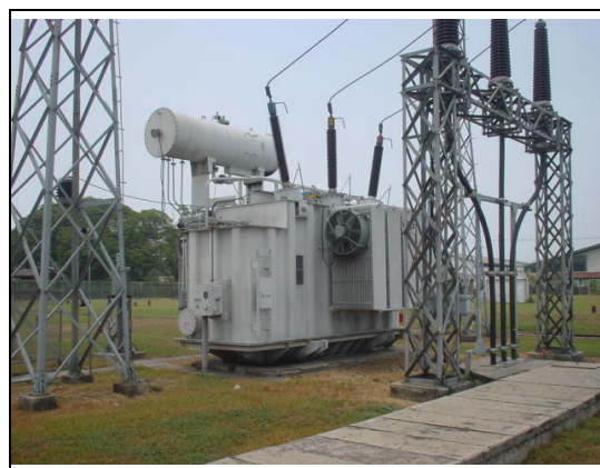
Substation installed via the project
