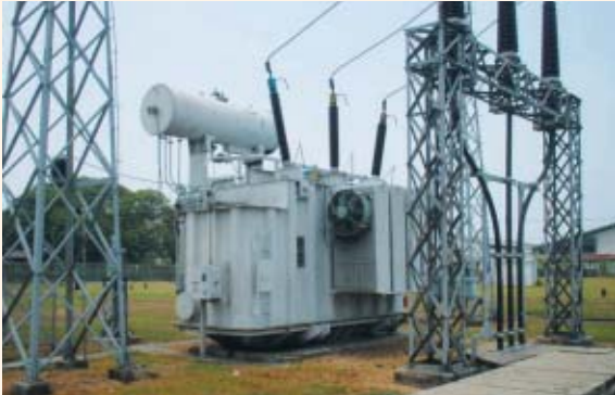
Substation installed by the project
