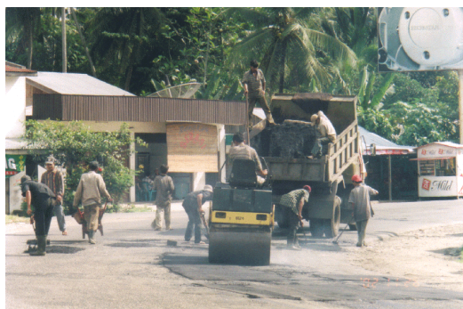
Maintenance work in progress on a national road (North Sumatra Province)
