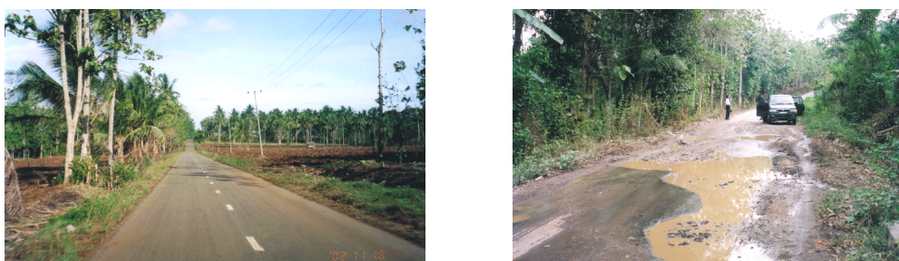
Figure 3: A section of road upgraded via the project (left) and a road connecting with the upgraded route (right: not covered)
