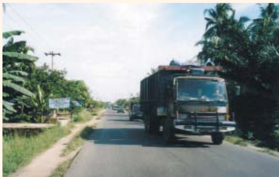
National road maintained through this project (North Sumatra Province)
