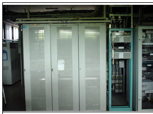
Optical transmission system installed in the course of the project
