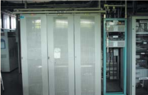
Optical transmission system installed through this project
