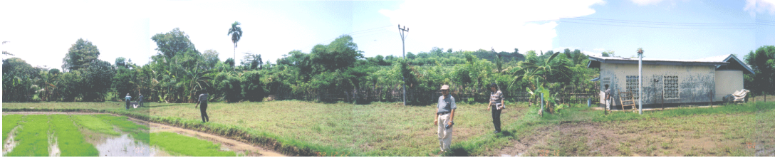
Figure 4: Beneficiary areas (A pump shelter on the right)
