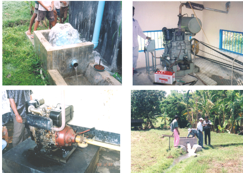
Figure 8: Pumps installed in the project and water springing from the distribution box
