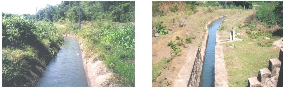
The secondary canal maintained by WUA (right) is better cleaned than the main canal maintained by the government (left)
