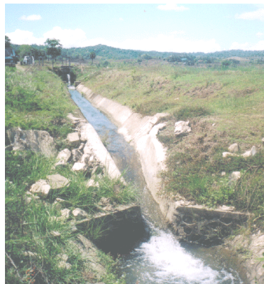
Figure 6: Drop structure on the secondary canal repaired by WUA
