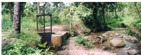
Figure 6: An example from Village Irrigation Schemes restored under the project
