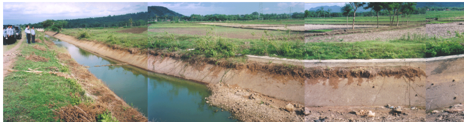
Figure 2: Primary channel sector where lining has been restored under the project
