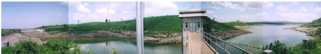
Figure 4: Sangiran Dam built under the project
