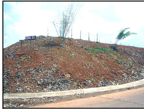
Figure 4: Condition of Completed Sanitary Landfill at the Final Disposal Site
