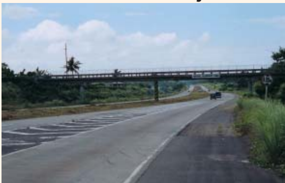
The expressway constructed via this project
