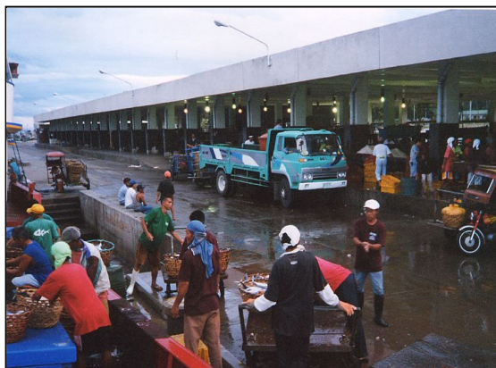
General Santos Fish Port Complex
