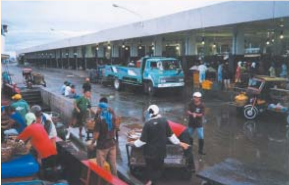
General Santos Fish Port Complex developed by this project
