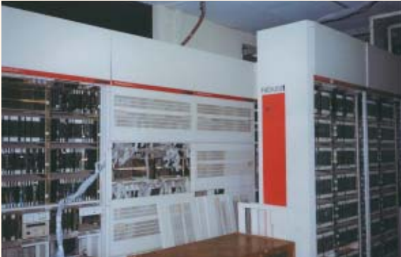
Switching facility installed by this project
