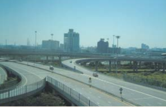
The expressway constructed under this project
