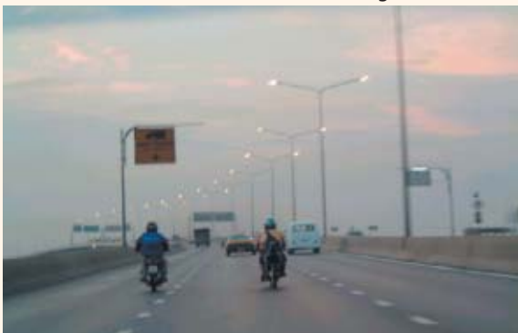
The New Krung Thep Bridge constructed under this project
