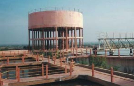
Purification plant constructed under this project (Solapur)
