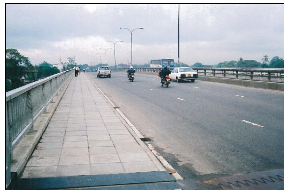
The New Sri Lanka - Japan Friendship Bridge constructed under the project
