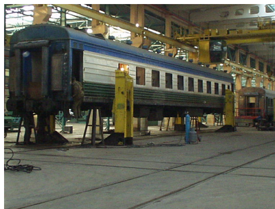
The passenger car repair shop constructed under the project
