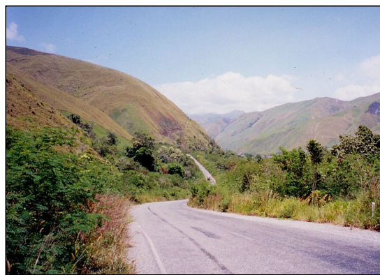
Road section: Mumeng-Bulolo
