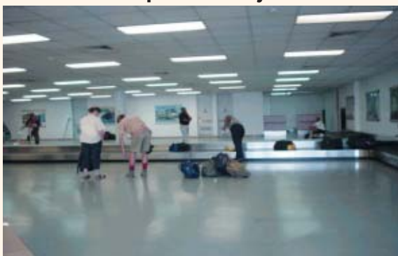
Domestic line baggage claim area installed by the project
