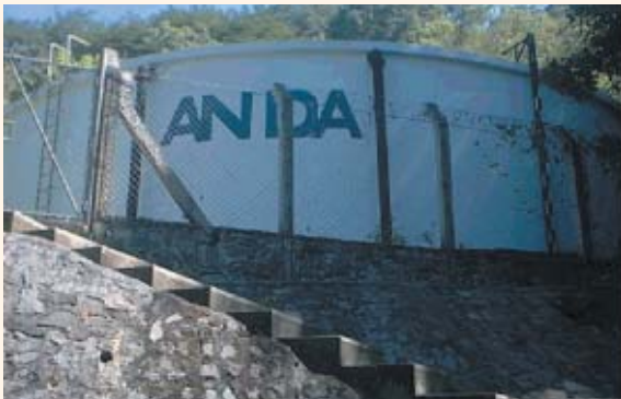
A water storage tank installed by this project
