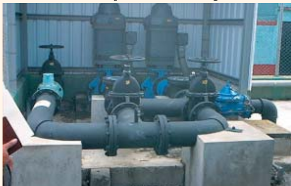
A deep well constructed under this project
