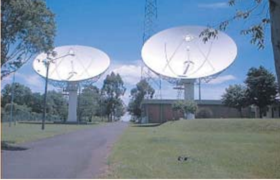
Parabola antennae installed by this project
