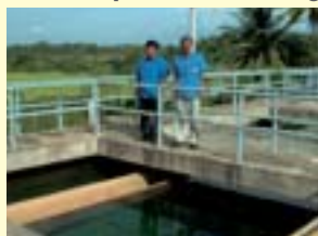
Filtration plant in Phattalung
