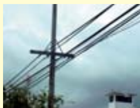
Cables in Trat Province (the thick central cable was installed by this project)
