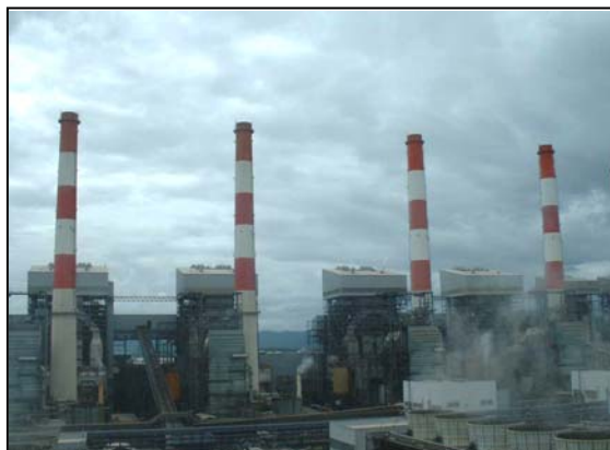
Generators 8 thru 11 where desulphurization equipment was installed
