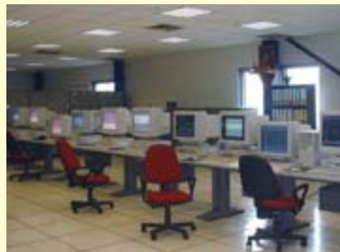
Having both domestic and abroad inspection parties to the flue gas desulfurization equipment control room to stimulate the technology.
