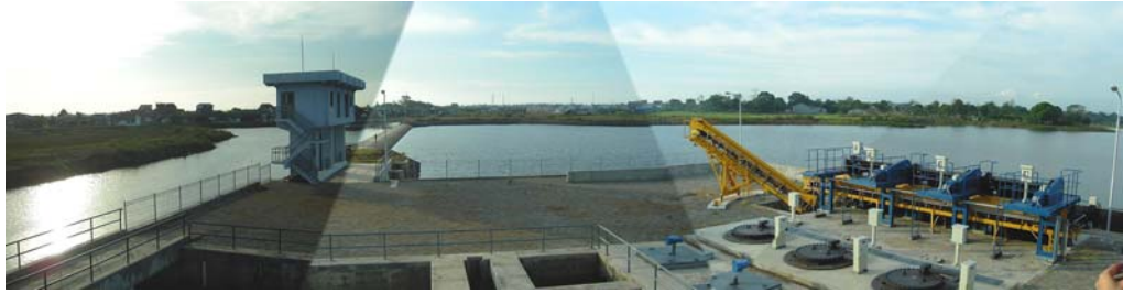
Figure 3: Pampang Regulating Pond
