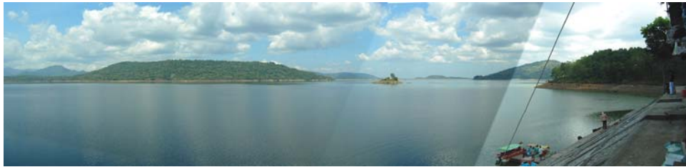
Figure 6: View of the Dam Reservoir
