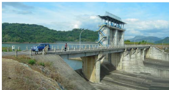
Bili-Bili Multipurpose Dam spillway
