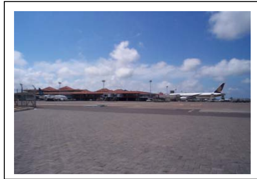
View of international apron / terminal from west side
