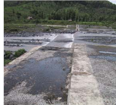
Consolidation dam on Mt. Semeru
