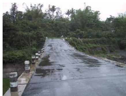
Figure 2: Check Dam on the Boyong River (headwaters are on the right)
