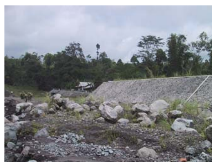
Figure 4: Training dike on Mujur River headwaters
