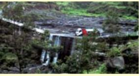
The debris flow that occurred in the Apu River in January 2003 completely filled the check dam. Had there been no check dam, the village located down river (Muntilan) could have sustained considerable damage. The debris flows that occurred on Mt. Merapi in 1992 and 1994 (10 million cubic meters) were approximately 2.5 times larger than that on Unzen-Fugendake volcano (Nagasaki, Japan) in 1993.
