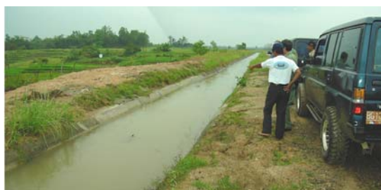
Figure 6: Examples of Rehabilitated Secondary Water Canals
