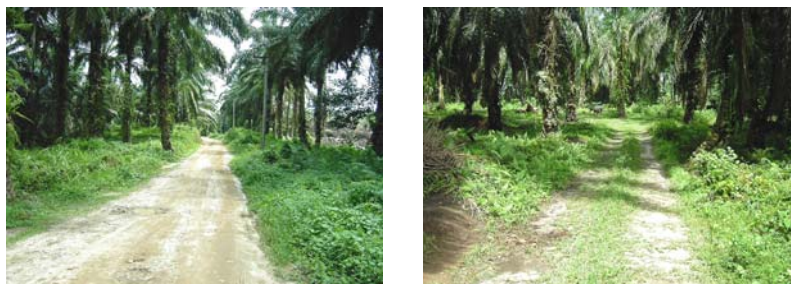
A production road feeding into a trunk road
